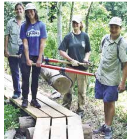
■ Bog Bridge construction.
